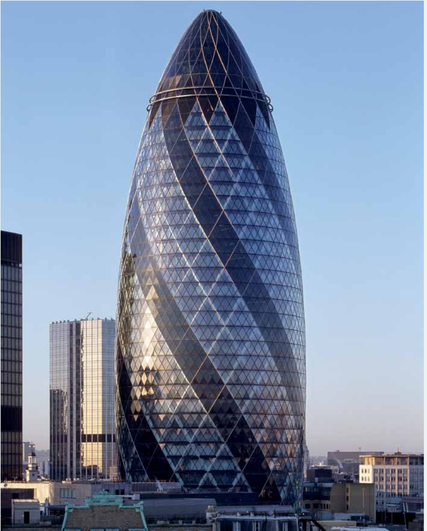
Swiss Re in London, 30 St Mary Axe. 2004, Architekt: Norman Foster.
